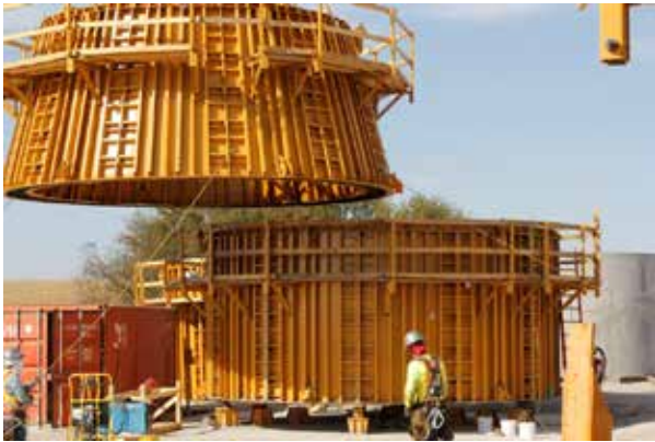
Formwork installed in precast yard to match-cast next segment
