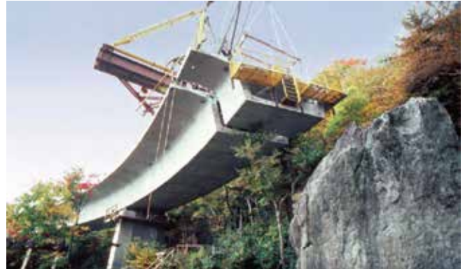
Precast segmental bridge construction using match-cast joints
