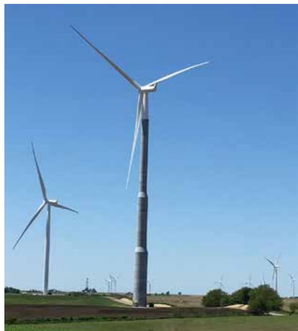
115 m precast concrete wind tower with 108 m (354 ft) rotor
