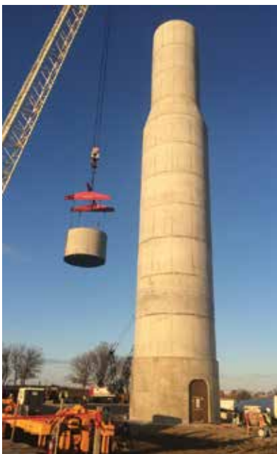
Precast segment lifted by crane for placement onto the tower
