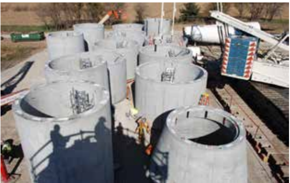
Finished segments in storage ready for installation into the tower
