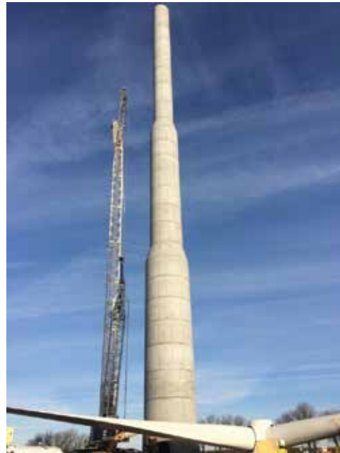
Precast segments fully stacked and post-tensioned to foundation
