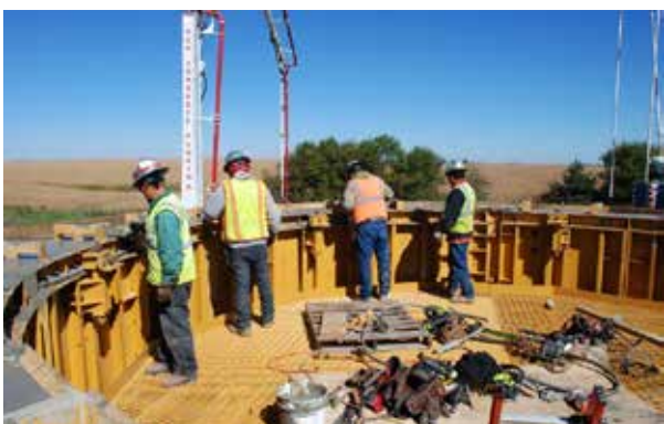
Concrete finishing of segment joint in preparation for next casting
