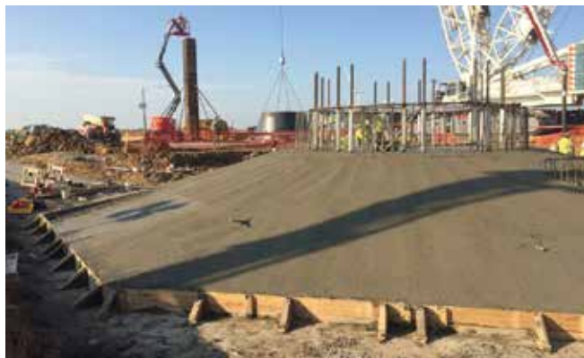
Cast-in-place foundation placed prior to casting pedestal wall and backfilling with soil
