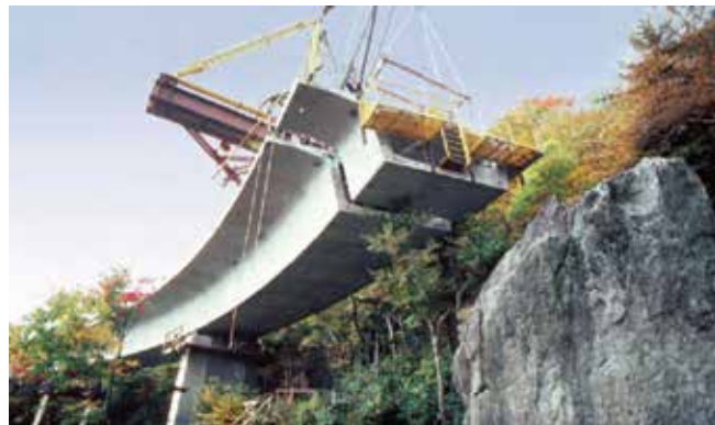
Precast segmental bridge construction using match-cast joints
