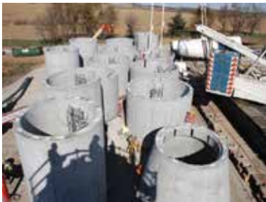
Fig. 3—Precast segments are match cast.
