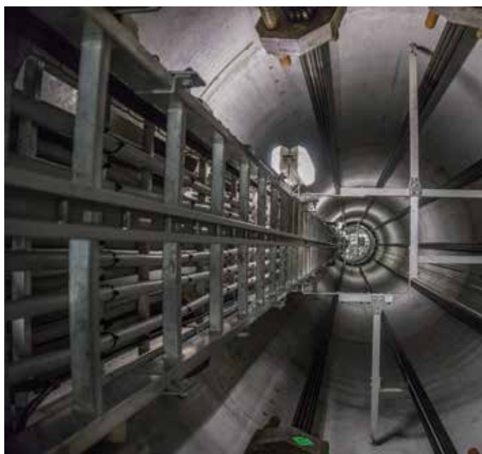
Fig. 7—Nineteen-strand external tendons around perimeter of tower.
