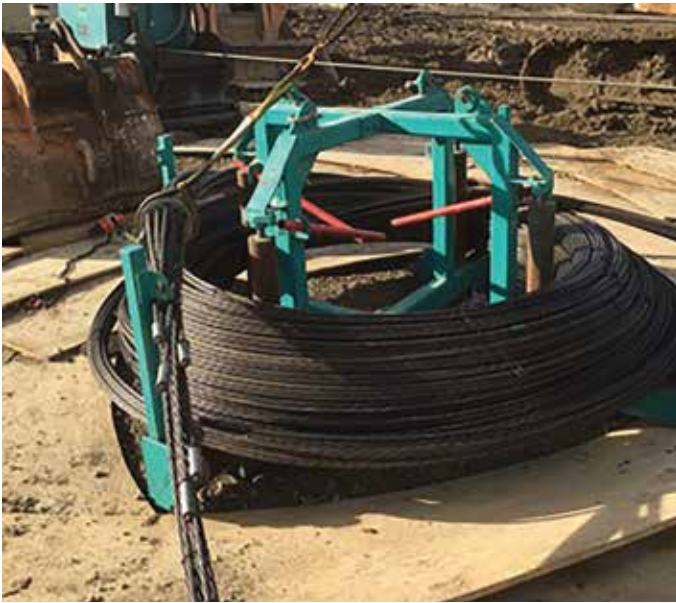
Fig. 8—Prefabricated tendons shipped to site ready for installation.
