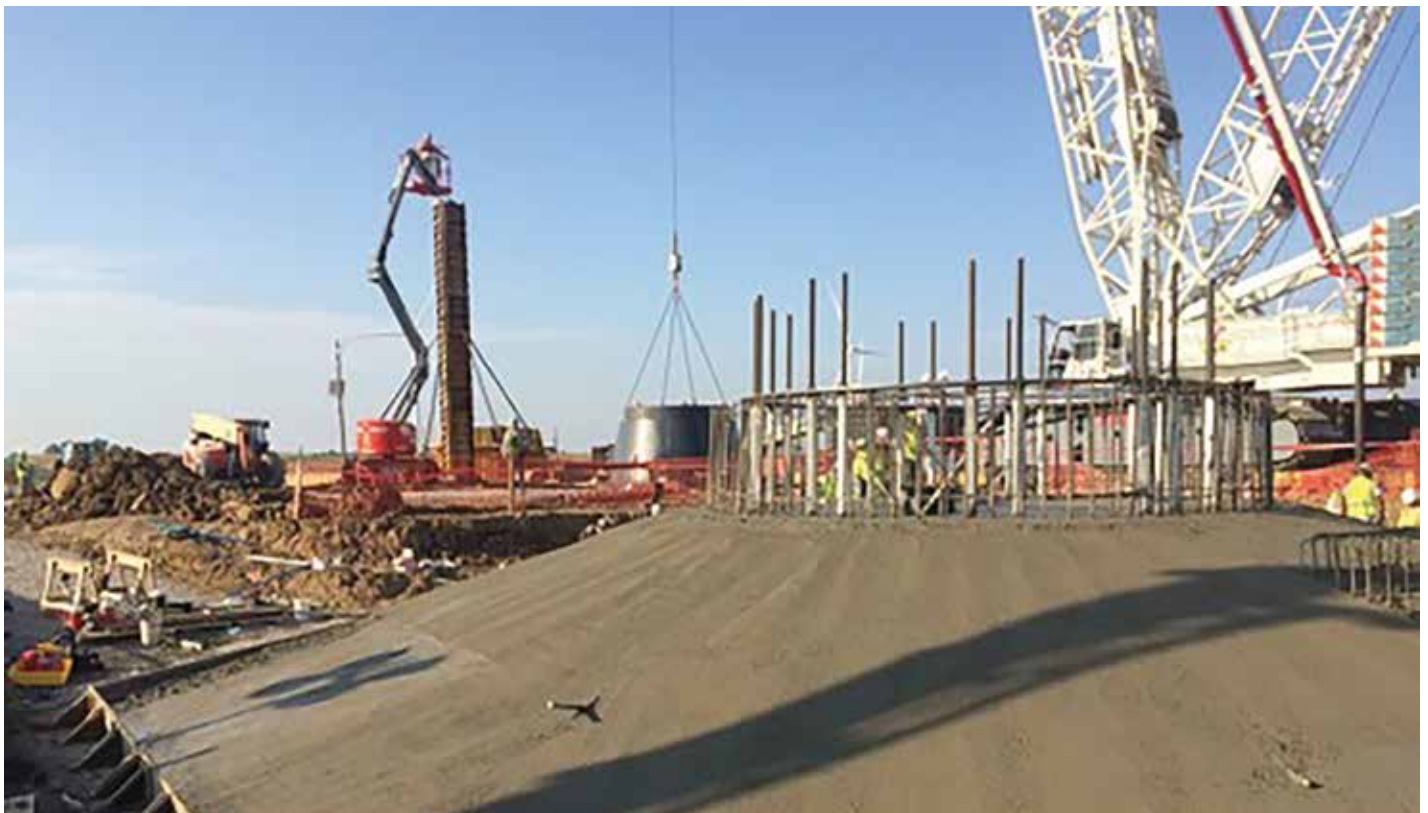
Fig. 4—Cast-in-place foundation.
