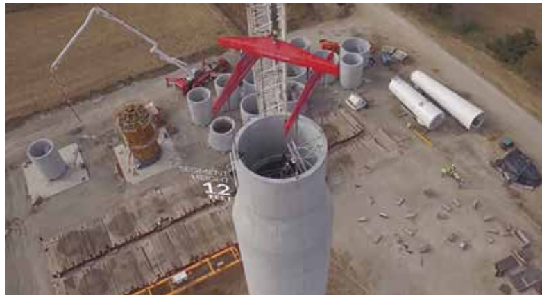
Fig. 6—Stepped concrete tower design.
