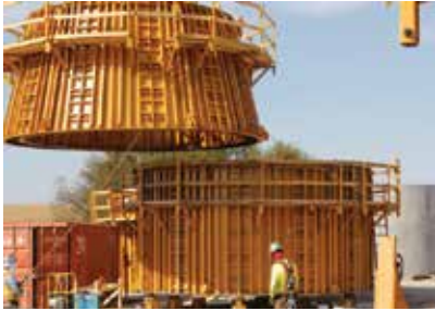
Fig. 2—On-site segment precasting.
